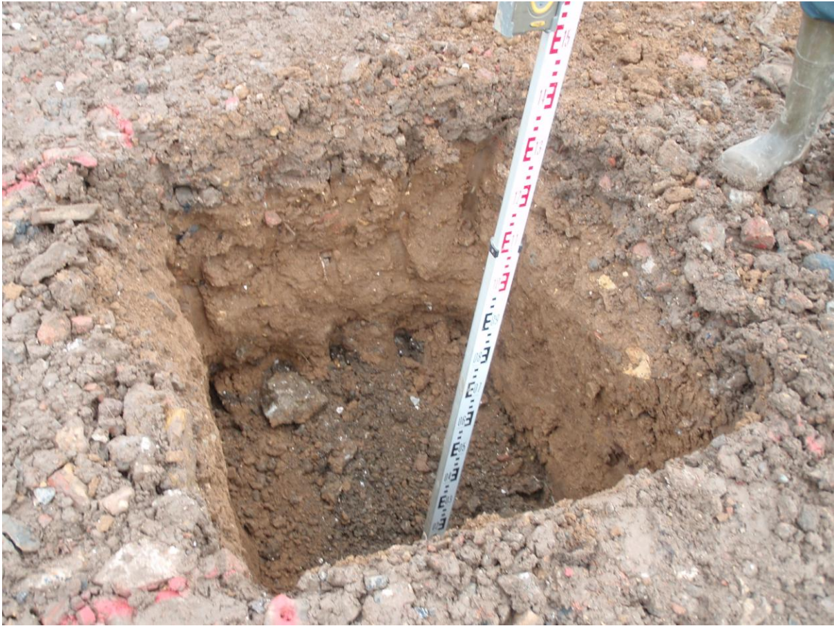
Plate 4. Foundation pad facing north
