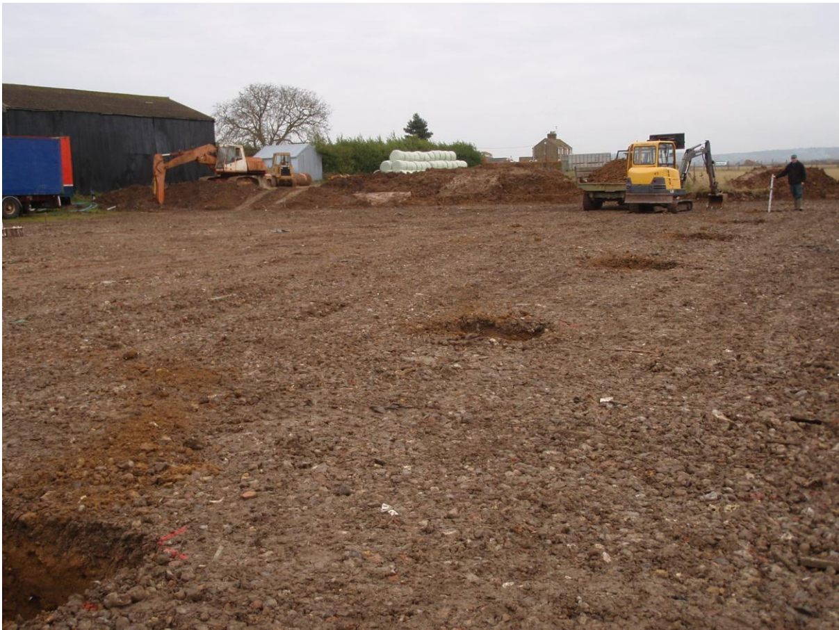
Plate 2. General view of site with post pads excavated, facing north-east
