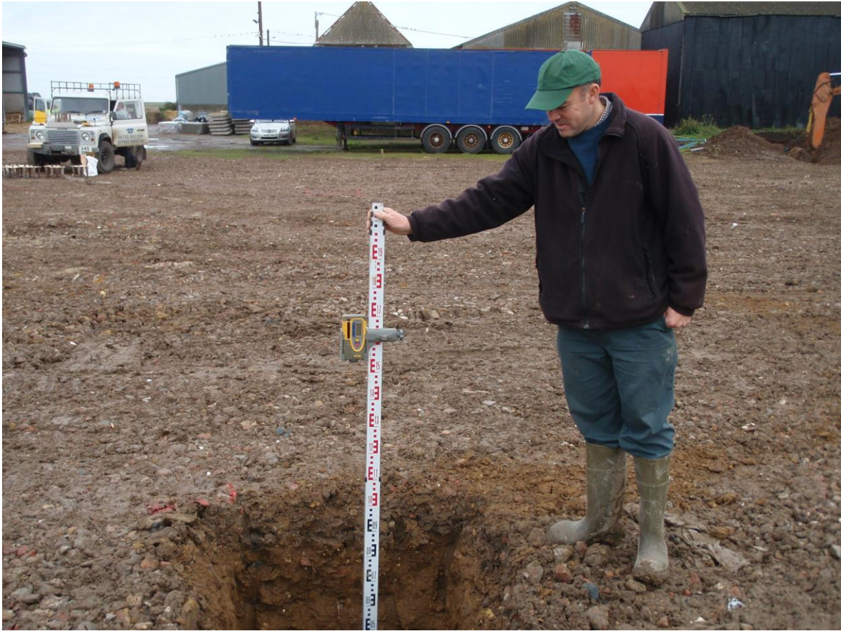
Plate 3. The site showing ground works (post pads) facing north
